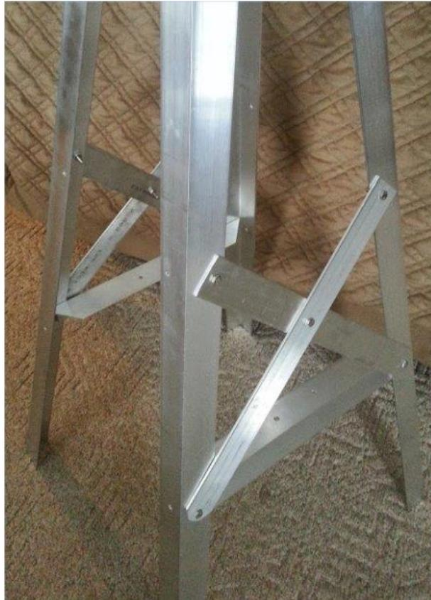
7. Attach the remaining 2 sets of X-braces on each of the 2 open sides as shown below, using 5/16"-18 x 1" bolts and locknuts. Spread the tower legs apart until the lower holes of the X-braces line up with the holes in the tower legs. Hand-tighten the upper set of bolts in these 2 assemblies at this time. See the image below.
